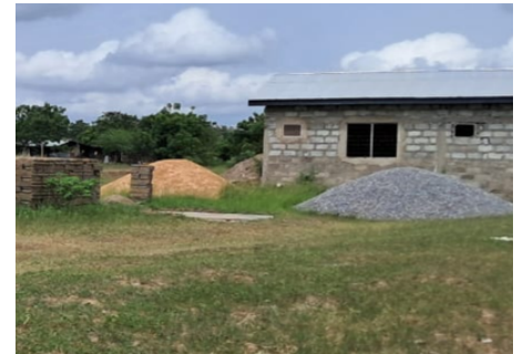
Ongoing construction around the reserve
